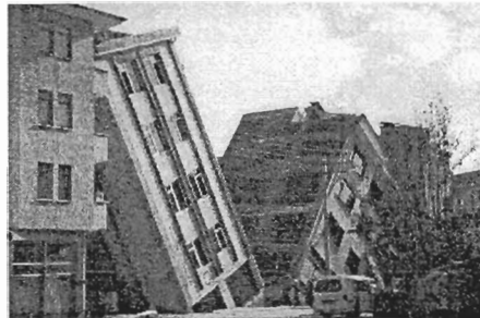
Figure 5 Bearing failure, Adapazari
